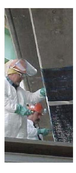
Repair any large areas of spalled, delaminated, or otherwise deteriorated areas of the concrete substrate and inject any existing cracks in the substrate. Profile the concrete surface by abrasive blasting, water blasting, or disc grinding.
