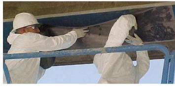
MBrace® can be applied to concrete and masonry walls to increase their resistance to out-of-plane loads. This includes loads due to wind, soil pressure, fluid pressure in tanks, and blast loading.
