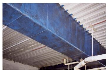
"U" wrapping — simply wrapping the sides and bottom of the section— can increase the shear strength of beams in high shear zones. An additional 1 to 2 kips (for every inch of beam depth) or 200 to 400 N (for every millimeter or beam depth) of shear capacity can be gained by "U" wrapping with MBrace® reinforcement.
