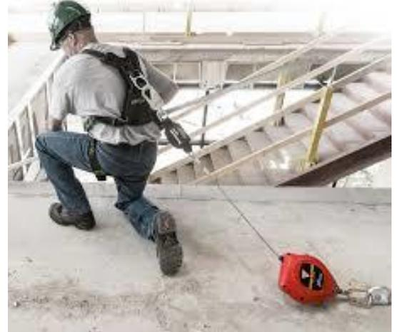
**TOP DECK WORK - The 30-50 ft retractable life-line is anchored to the wall and laid on the deck. The line is connected to the worker’s retractable lanyard. The retractable life-line is locked so that the worker cannot fall over the edge. This will require constant monitoring and adjustment as the leading edge moves.**
