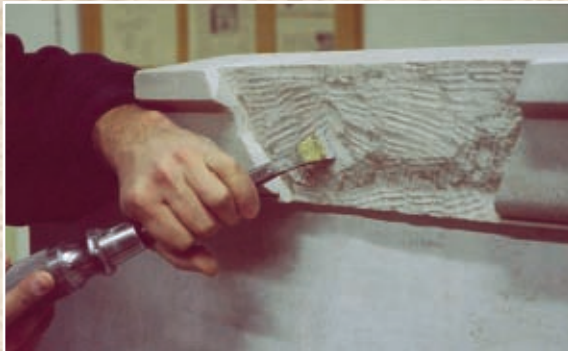
Incorrect ( Feathered Edge ) Surface Preparation
